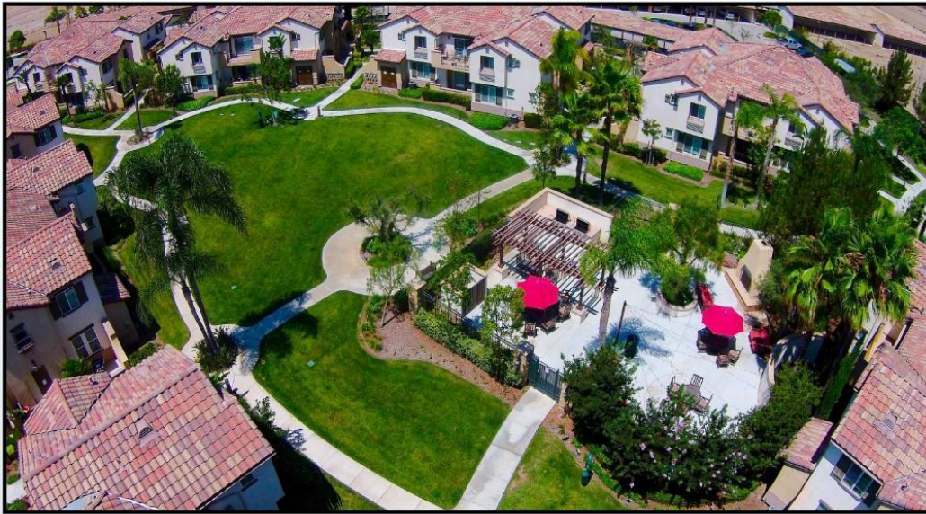
Villas at the Park, a luxury apartment community in Camarillo, CA purchased in March, 2015.
